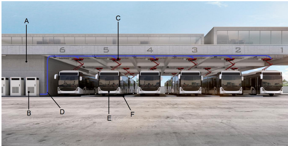
Example of a complete installation
