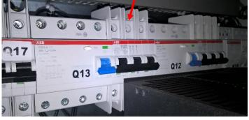
8) After opening the door, identify and switch off Q12, Q13, and Q17 which are located on the top-left side inside the power cabinet
