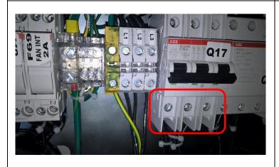
3) Measure on the Bottom terminals of Q17 to verify the power is switched off. The terminals are directly linked to the top side of the main disconnect switch.
