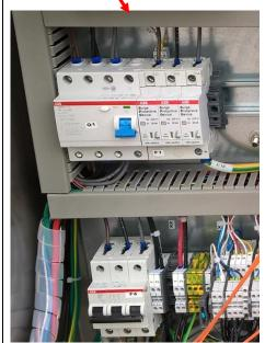
After opening the door, identify and switch off F4 and Q1 which are located on the left side inside the ACM.
